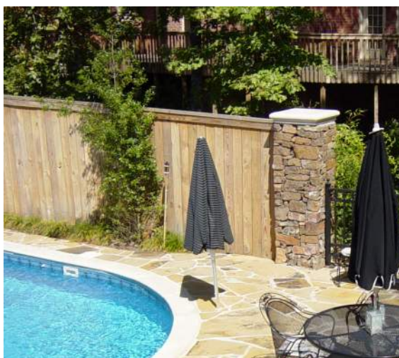
Fencing must have a top rail and post in residential applications.
